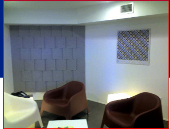
Worrell used the 8" round BAP Blade to cut the panels into 1 x 1 squares and installed them in an alternating overlapping pattern.
