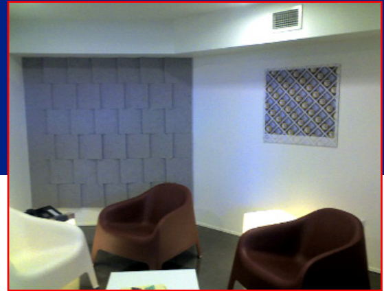
Worrell used the 8" round BAP Blade to cut the panels into 1 x 1 squares and installed them in an alternating overlapping pattern.
