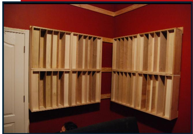
*The installers field fabricated some Schroeder diffusers to help create a balanced and full sound in the small studio.*
