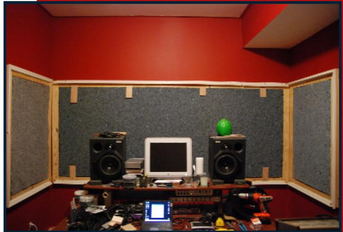
*The Echo Eliminator was adhered to the wall with a construction adhesive. For this installation, the installers used some wood scraps to hold the panels in place – these were temporary to hold the panels until the adhesive dried.*
