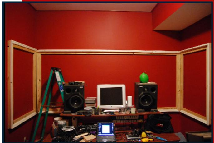
*The picture above shows the Wallmate track installed on top of the 1" thick furring strips. This allowed the owner to use the 2" thick recycled cotton panels to achieve a desired result. The 2" thick panels have a better low-frequency response with regard to the 1" thick panels that are considered "standard".*
