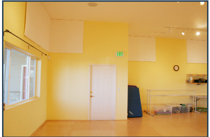
The acoustical paneling used in these rooms was our 1" thick, #3 lb. Echo Eliminator in white.
