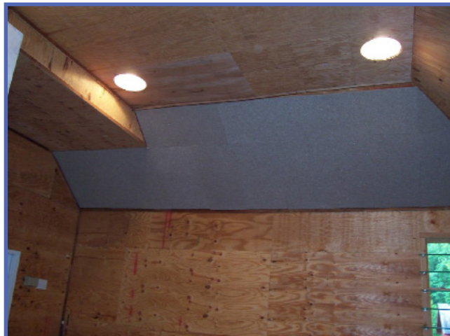
To install the panels, the installers used a combination of spray (contact) adhesive (AGS-12) as well as a construction grade adhesive (PSA-29). The contact spray adhesive grabbed right away and gave the construction adhesive time to set-up.
