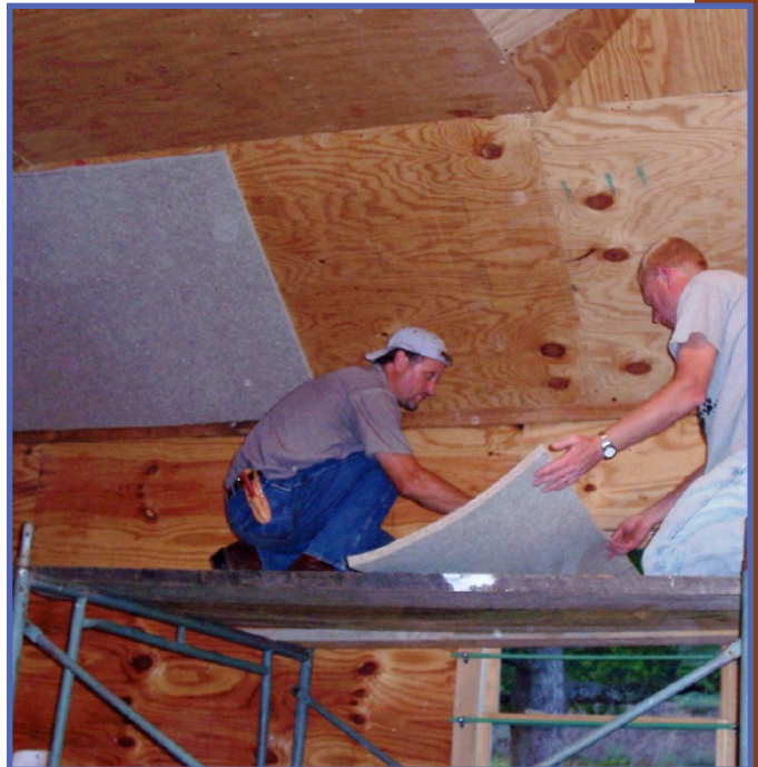
To install the panels, the installers used a combination of spray (contact) adhesive (AGS-12) as well as a construction grade adhesive (PSA-29). The contact spray adhesive grabbed right away and gave the construction adhesive time to set-up.
