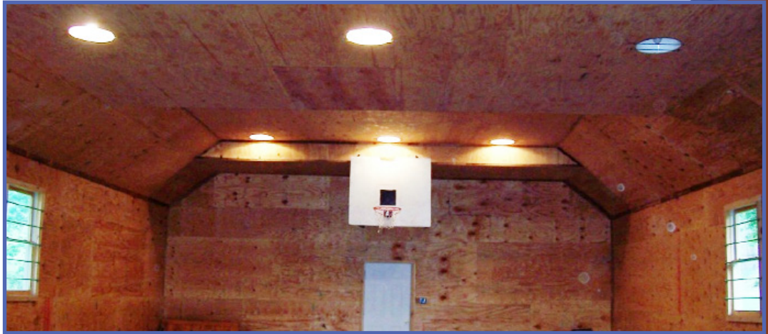
This plywood room had a reverberation time that would not allow it to be used for recreation and instruction at the same time. The church needed a cost effective way to remove the echo. 1" thick, Echo Eliminator panels were installed and dramatically reduced the echo.
